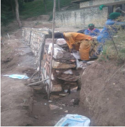
Building the drainage and fence retaining wall
